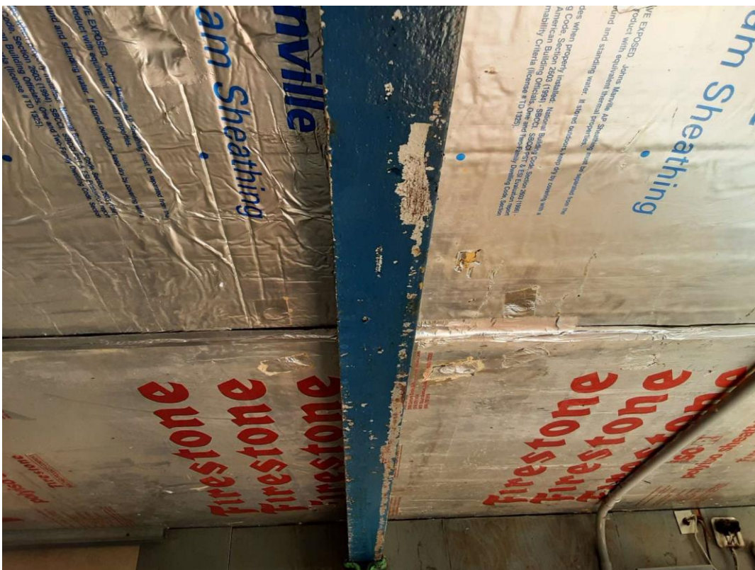
Metal, Blue over silver, L0003(Lead-containing), Control Room (Location #: 1)
