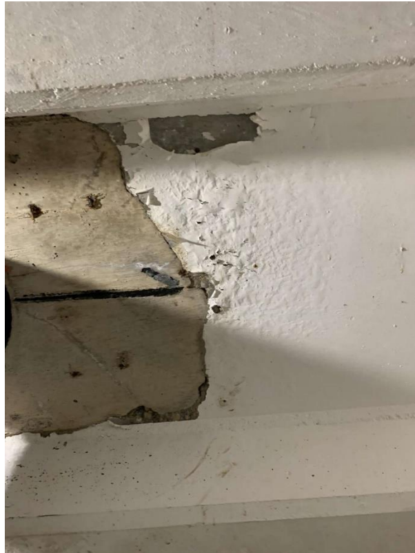
Concrete (poured), White, L0008 (None), Pump Room (Location #: 5)
