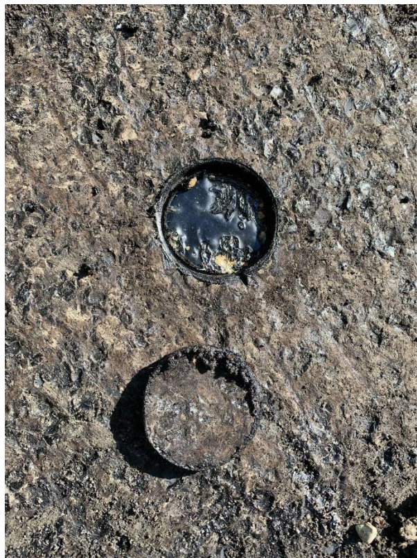
S0001B (None), Roofing material, Roof (Location #: 7)
