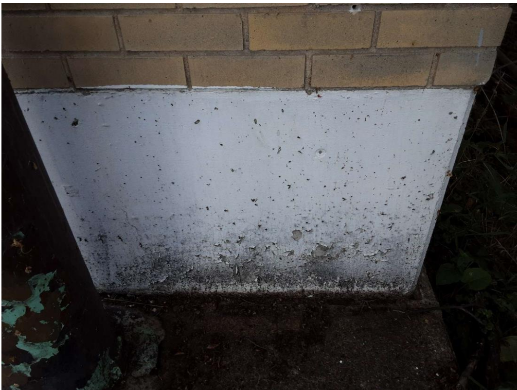
Concrete (poured), White, L0001(None), Exterior of Building (Location #: 6)
