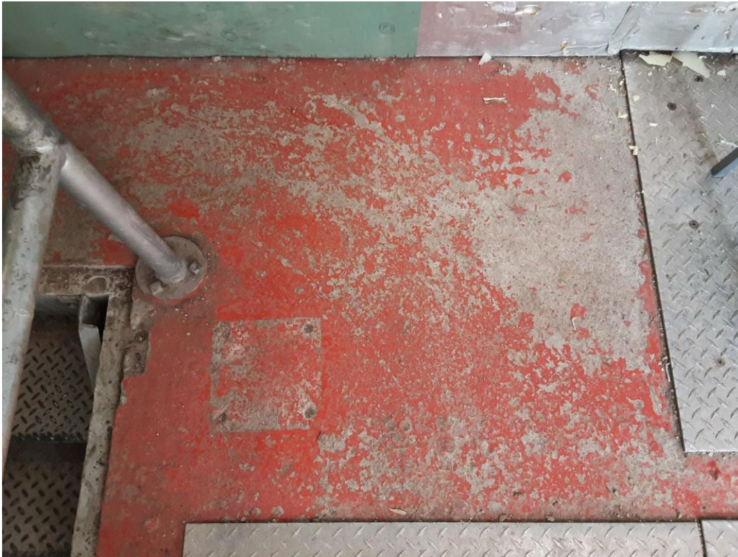
Concrete (poured), Red, L0004(Lead-containing), Control Room (Location #: 1)
