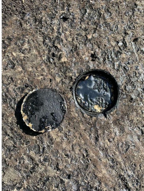
S0001A (None), Roofing material, Roof (Location #: 7)
