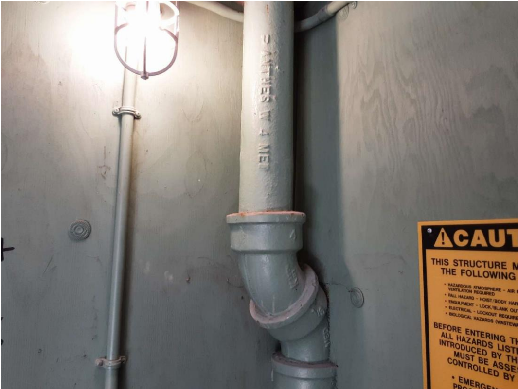
Metal, Green over silver, L0006(Lead-containing), Control Room (Location #: 1)
