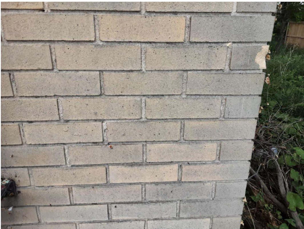
S0002A (None), Wall, All, Plaster, Exterior of Building (Location #: 6)
