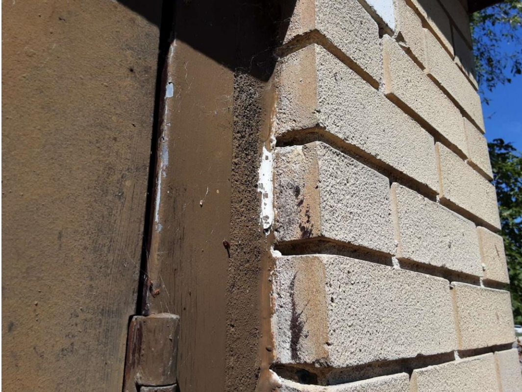
PCB (Non-PCB), Exterior of Building (Location #: 6)
