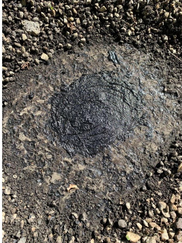
S0001C (None), Roofing material, Roof (Location #: 7)
