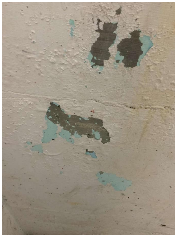
Concrete (poured), White over blue, L0007(None), Pump Room (Location #: 5)
