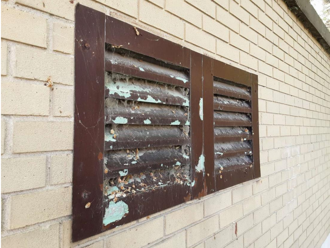
Metal, Brown over grey, L0002(Lead-containing), Exterior of Building (Location #: 6)
